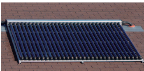
Solar thermal tubes supplying plentiful hot water
