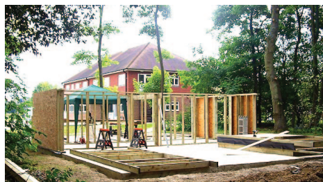
Complete on-site construction, no prefabricated sections.
